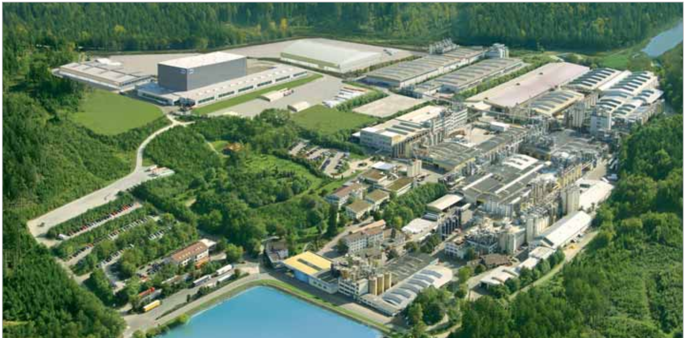
JRS Company Headquarters, Rosenberg Plant (Germany)
