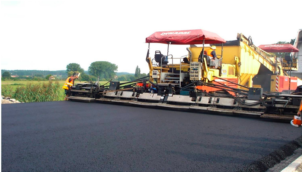
Figure 2, Laying of a SMA binder course
